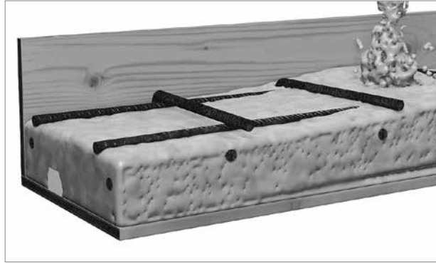
5. Concrete in the profile.
